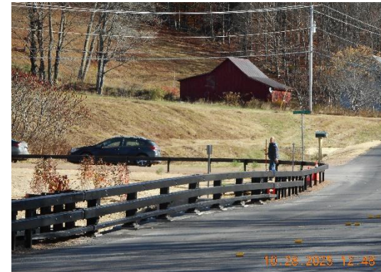
Example of Powder Coated Bridge Rail
